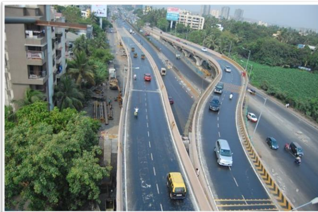
Amar Mahal Flyover
