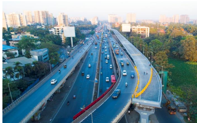
Chheda Nagar Flyover Part 1
