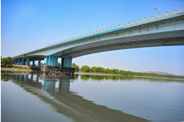
Motagaon Creek Bridge
