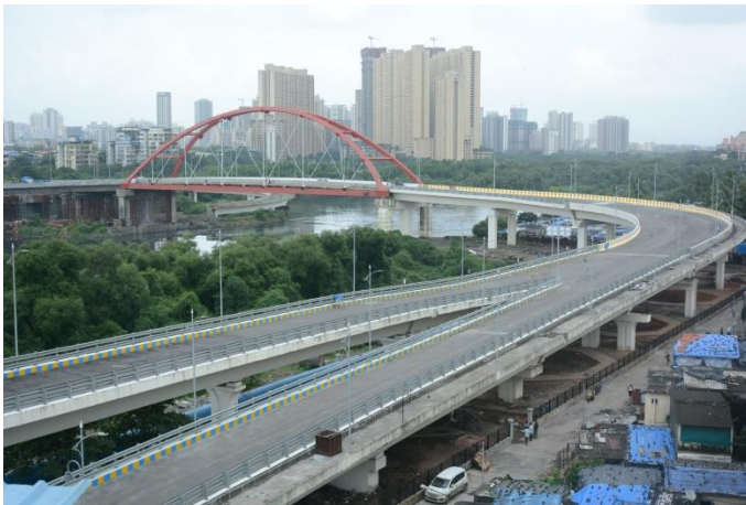
Kalwa Bridge Thane
