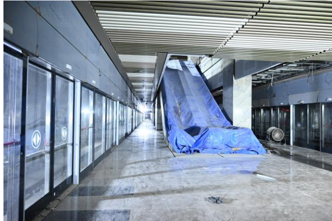
Mumbai Underground Metro Line 3
